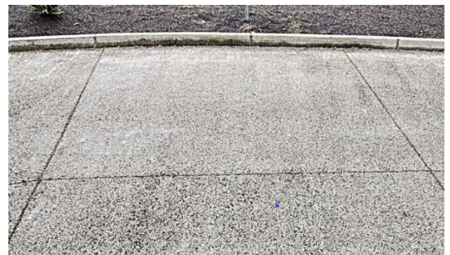
This area was treated with baking soda 10 months prior to the photo and the moss has not grown back.
