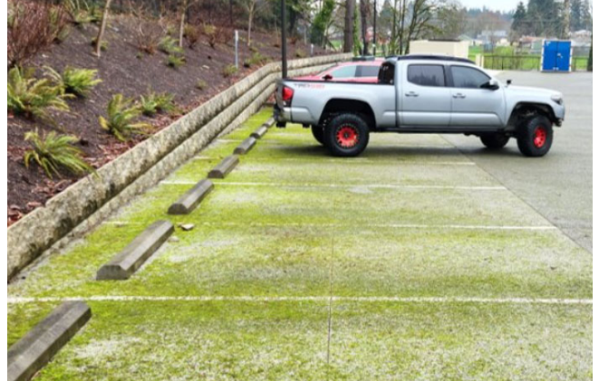
This 5-year-old pervious concrete is located next to a dense forest with heavy debris during winter. Because it was only maintained by leaf blowing, a lot of moss has built up. It's important to take steps to prevent this from happening.
