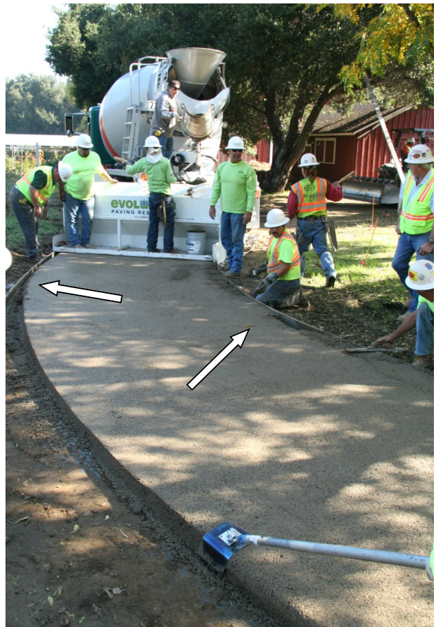
Measure pavement width in corners. Use 1 x board to straighten and fill edges to specified dimension.
